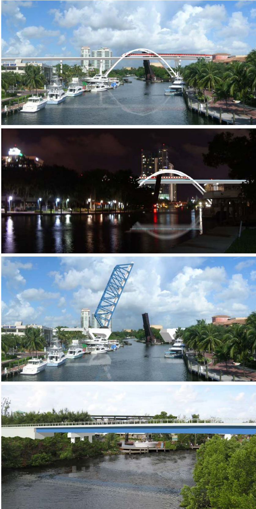
Figure 2.11 – Bridge renderings concepts - from top: New River high-level fixed by day; by night; New River mid-level bascule; Hillsboro River Canal
