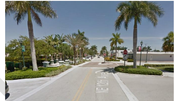
Phase I will require the removal of the island and repavement of the intersection and roadway. Photo Source: Google Earth
